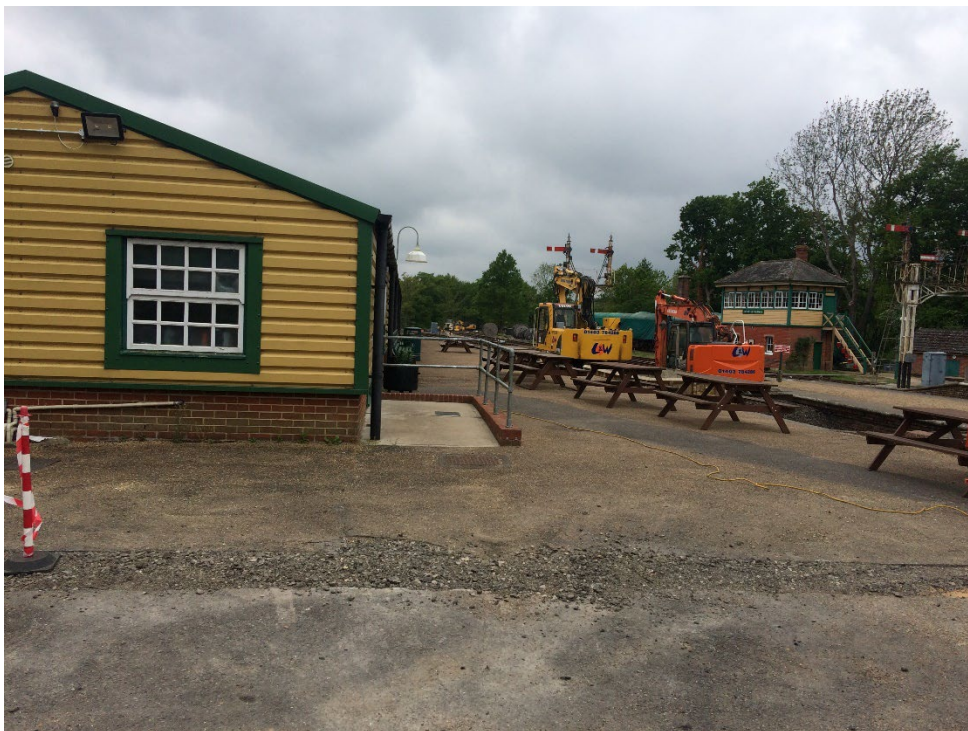
View towards Carriage sheds
