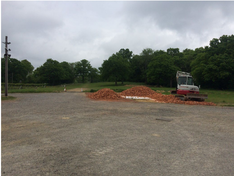
Further view of car park
